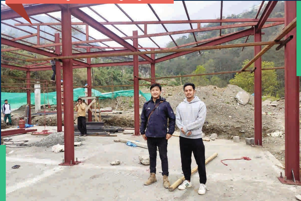
PHOTO37: Inspection of under construction craft beverage at Reshithang Gangtok.
