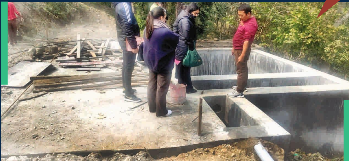
PHOTO34: Inspection of under construction ETP at the modern abattoir Melli.
