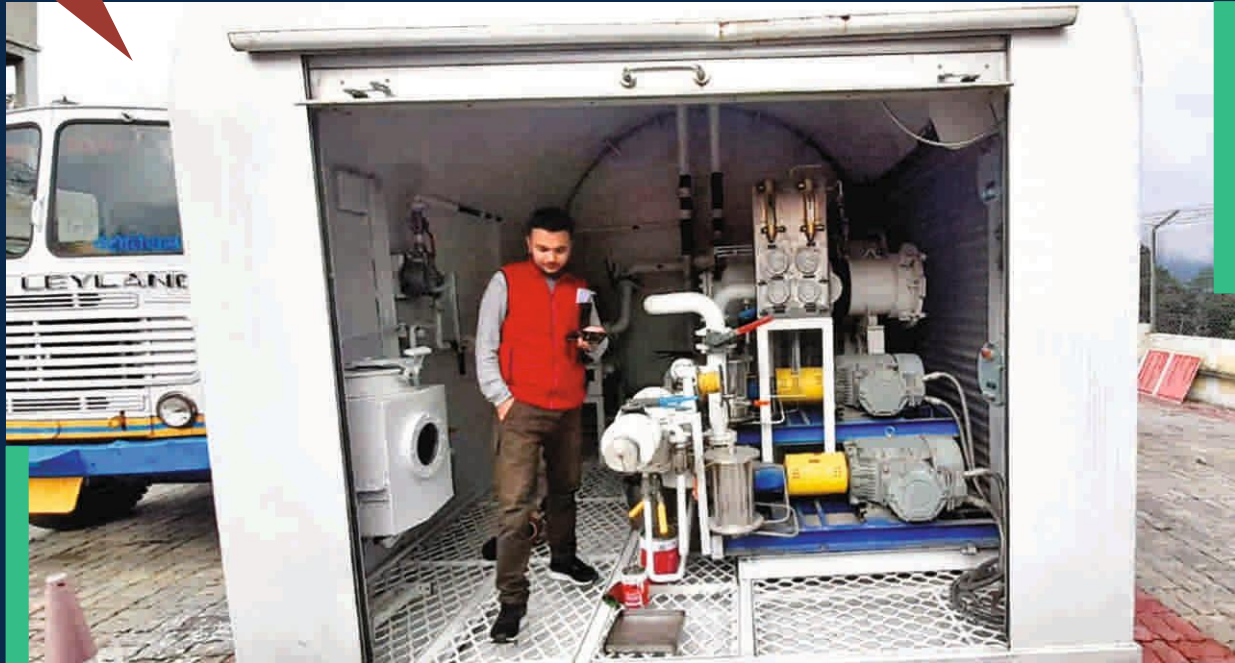
PHOTO33: Inspection of Oil Depot at Pakyong Airport.
