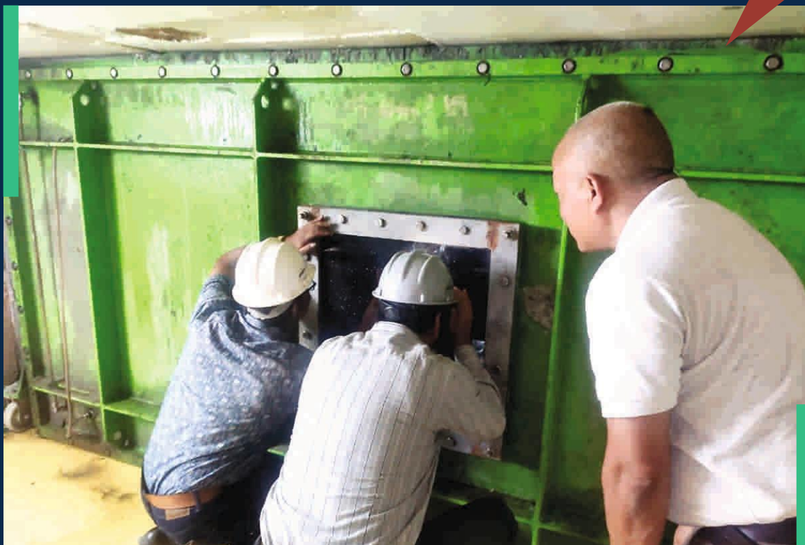
PHOTO35: Inspection of powerhouse site of MBPCL.
