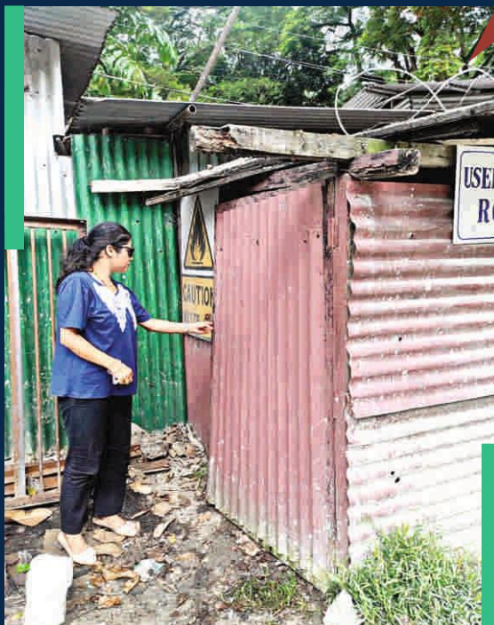
PHOTO45: Inspection of used oil storage room.
